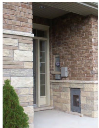
Utility meters should be recessed and hidden from view.
