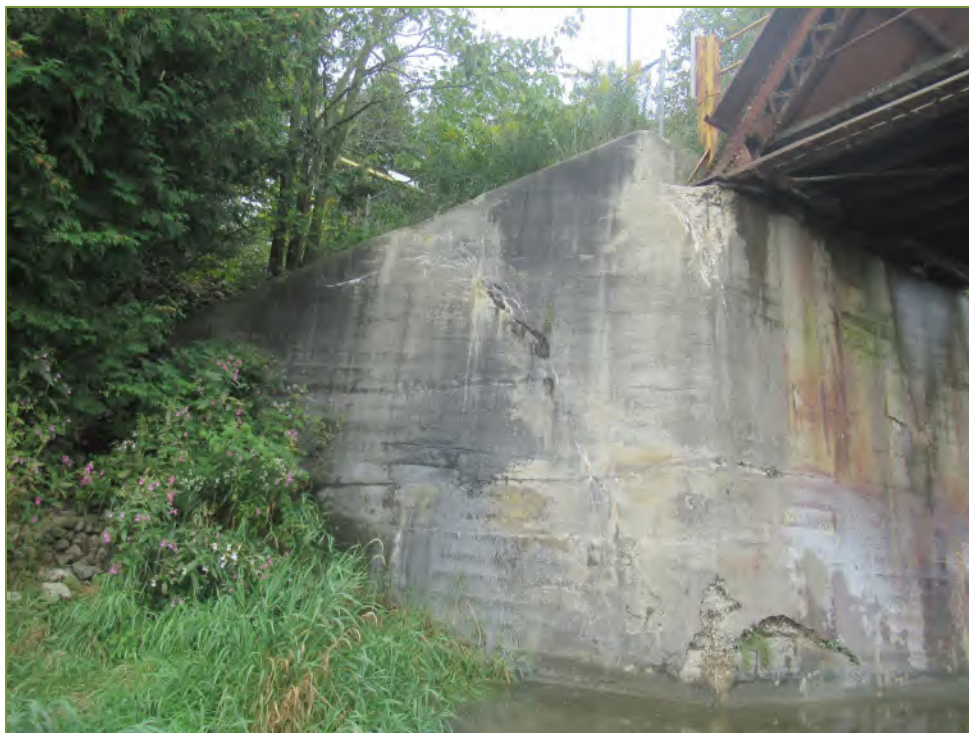
Photo P6 SW Wingwall
