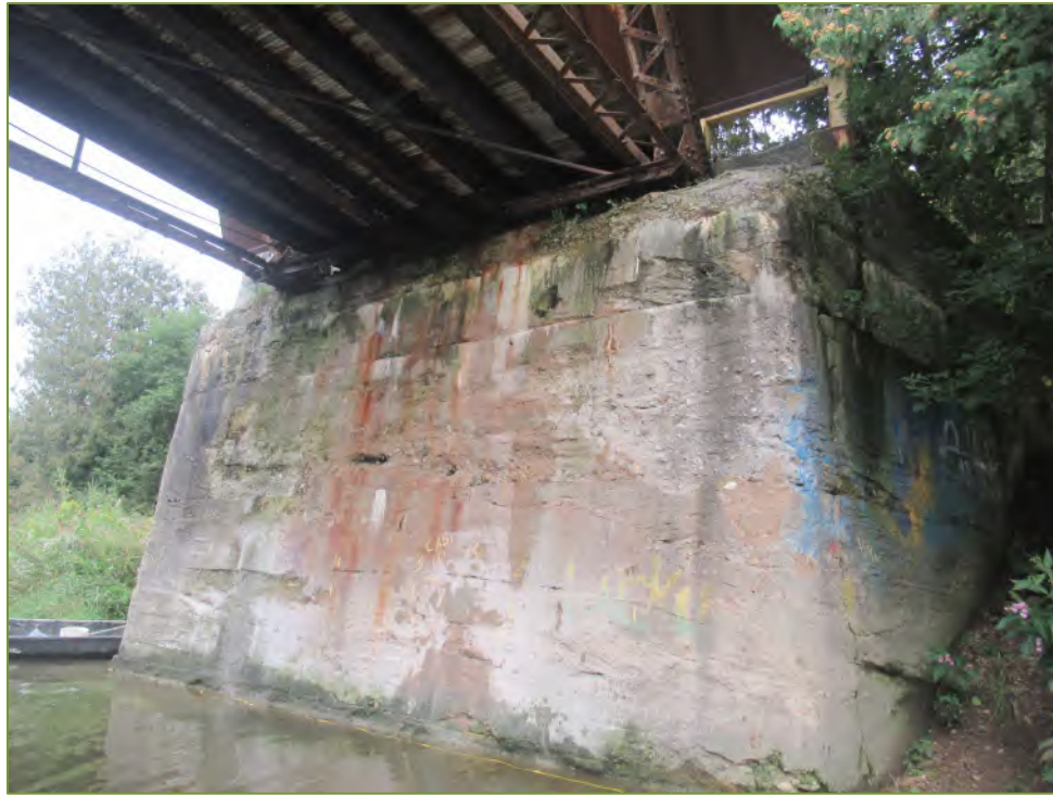
Photo P1 East Abutment
