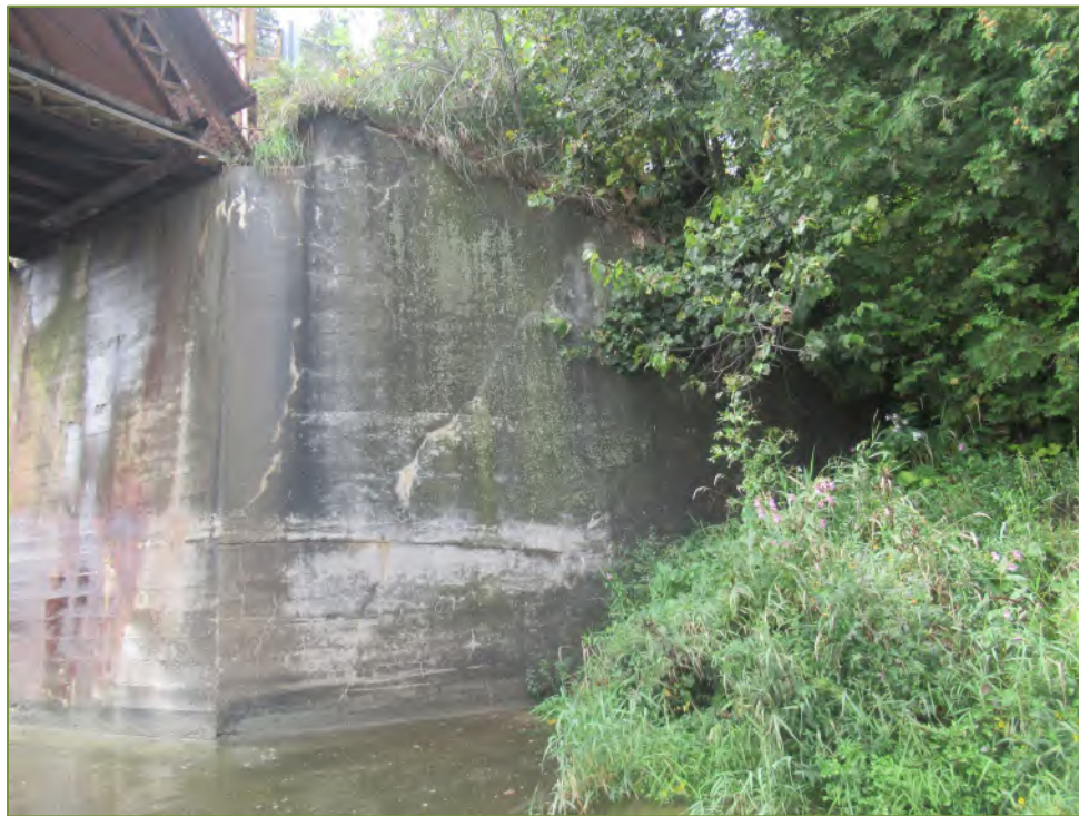
Photo P4 NW Wingwall
