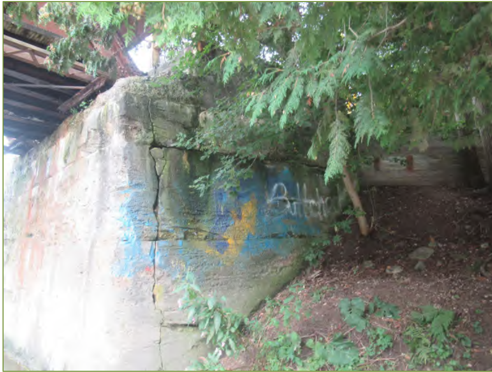
Photo P5 SE Wingwall
