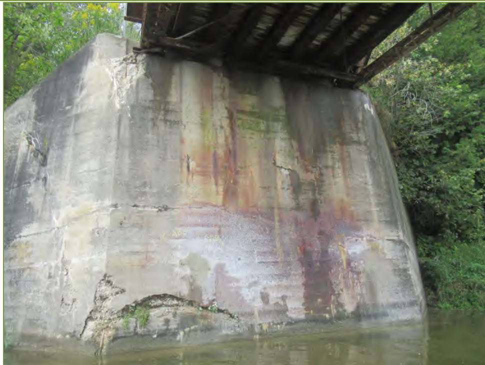
Photo P2 West Abutment
