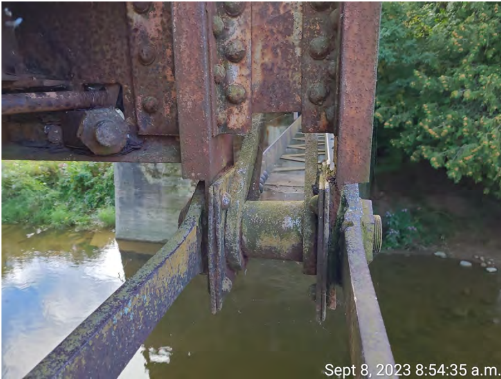
Photograph 11: South truss, Joint 3 showing medium corrosion of vertical web plates and gouge in exterior bottom chord.
