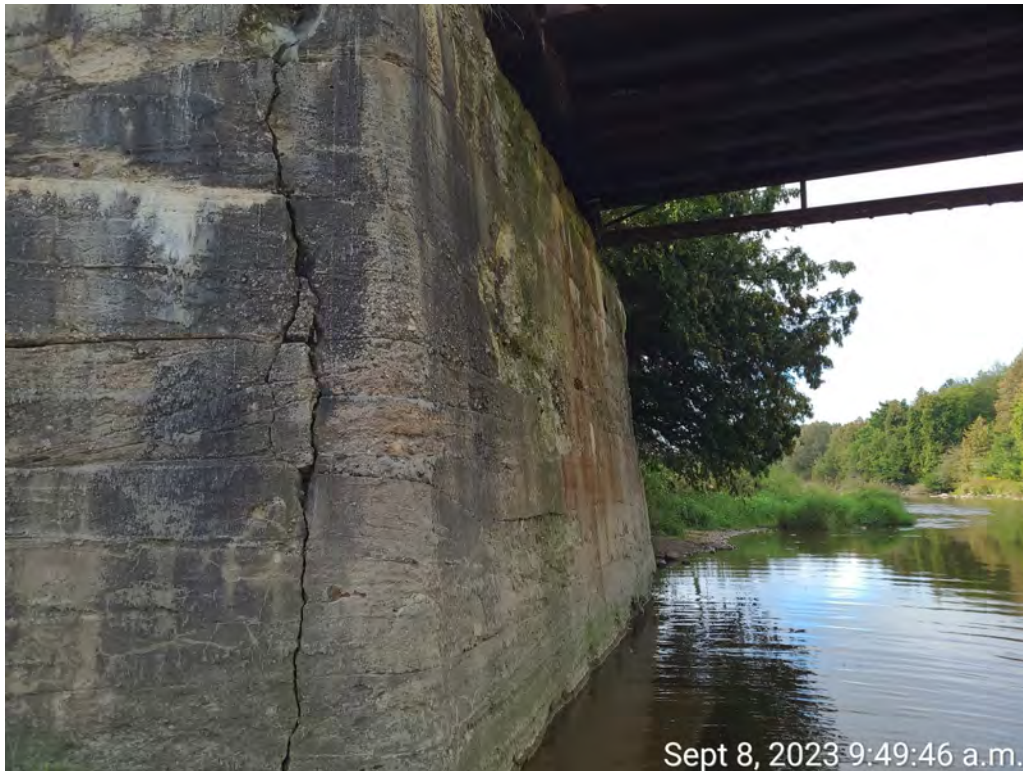
Photograph 18: East abutment, north wingwall showing wide vertical crack at wingwall/abutment interface. Footing repair visible below waterline.
