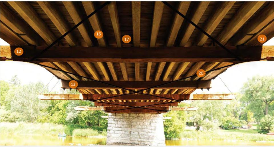
New Douglas Fir 16"x16" needle beams
