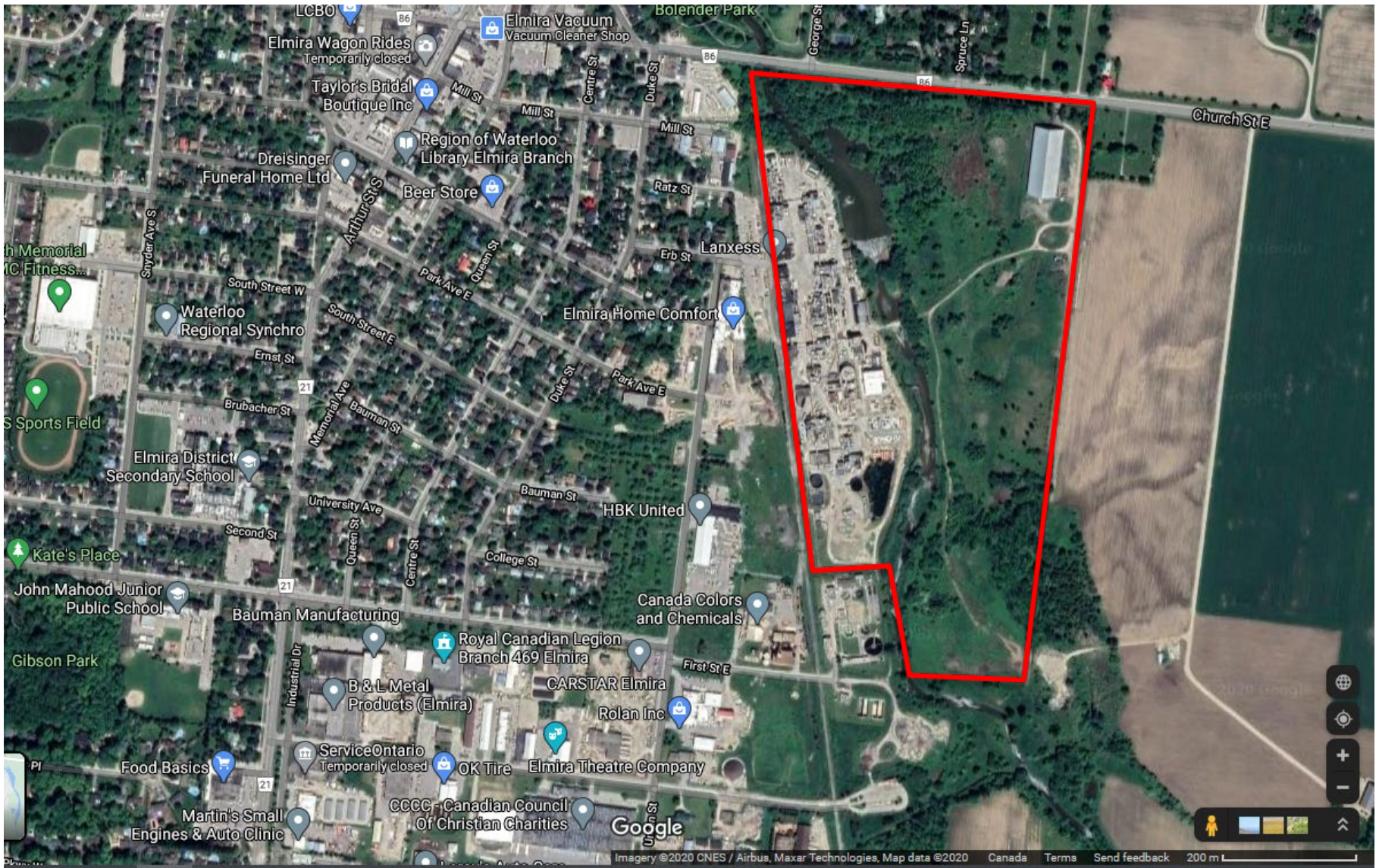
Current – Post Remediation of Historical On-Site Waste Management Units
