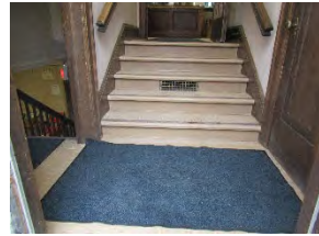
3 SJL - Stairs to main level
