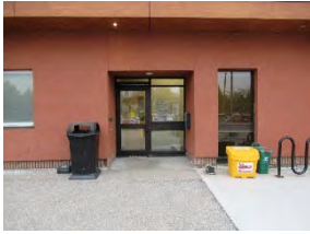
1 Woolwich Administration Office staff entrance
