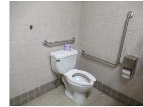
6 FFS - Mens washroom stall toilet area
