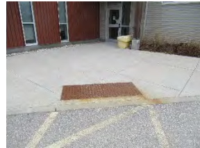
3 BFS - tactile warning plates 2
