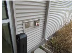
4 BFS - entrance controls
