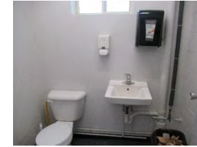
6 STJW - Mens washroom sink area
