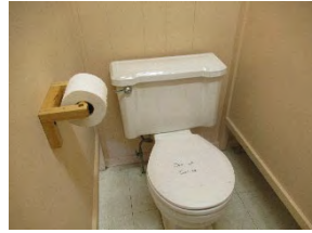
4 CCC Washroom toilet area
