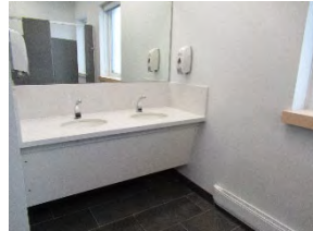
11 WAO Mens washroom sink area
