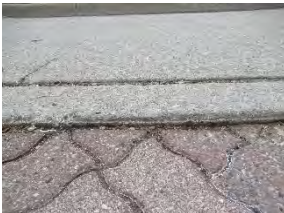
15 EL - first ramp - lip at entrance
