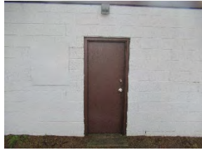
2 SPW - Washroom door
