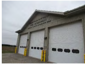
2 FFS - Bay doors
