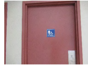
5 FFS - Mens washroom door
