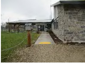
1 Heidelberg Community Centre entrance
