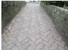
16 EL - first ramp surface
