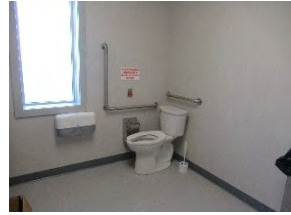
3 MFS Universal washroom toilet area
