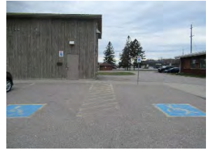
7 BS Accessible Parking
