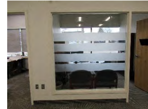
12 WAO office area window glazing
