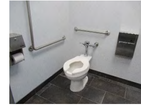
6 WAO Womens Washroom stall area
