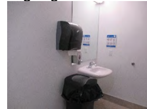
19 BFS Womens Changeroom washroom sink area
