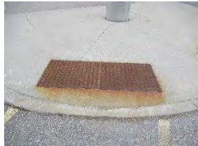
2 BFS - tactile warning plates
